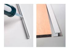
Apply RESOPAL SpaStyling connection adhesive to RESOPAL SpaStyling Connection Profile (H profile) profile openings ensuring precise application. Then the profile should be pressed against the long side of the RESOPAL SpaStyling BOARD. It is essential for the joint between profile and RESOPAL SpaStyling Board to be water-proof. Any RESOPAL SpaStyling connection adhesive oozing out from the profiles must be removed from the surface immediately.
