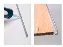
Apply RESOPAL SpaStyling connection adhesive to the inside of the RESOPAL SpaStyling end profile (L profile) ensuring precise application.
